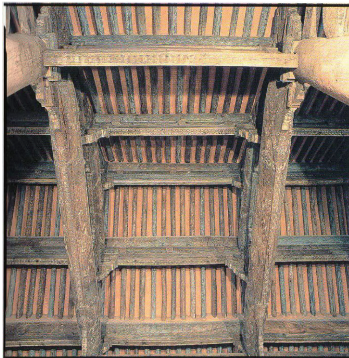
Figure 6. Internal structure of Sudeoksa Daeungjeon Hall
